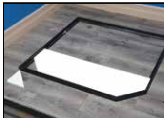
6. Lay in the Micore 300 triangle piece.
