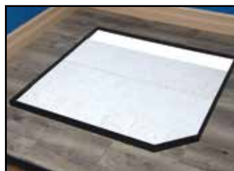
11. Lay in the remaining 12" x 36" Cement Board rectangle piece.
