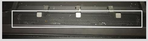
Place a thick layer of the ember glass over the perforations making sure to cover all of the holes completely.
